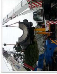
Seating the Exist LP Lower Casing
