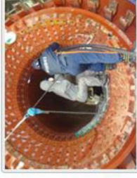
Blade Ring Dismantling, Lifting
